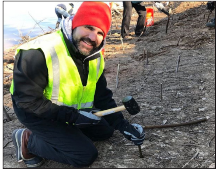
A planting of willow stakes along a streambank
